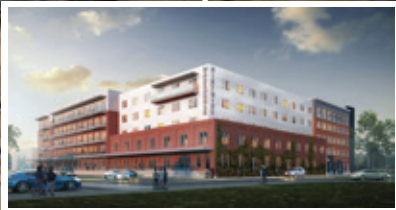
WAREHOUSE DISTRICT RE-DEVELOPMENT 800 BLOCK, WILLIAMS @ McKEE ST
