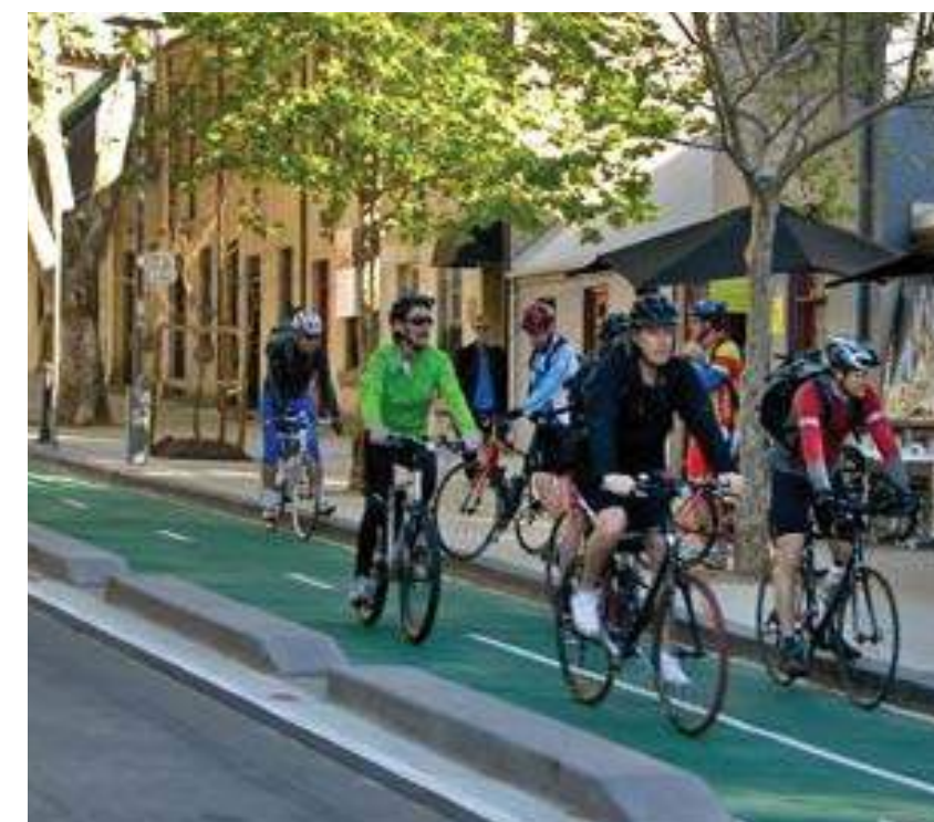
009 concrete bike lane delineators at intersection
