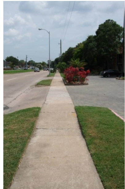
Example of Score 1, Good Condition
