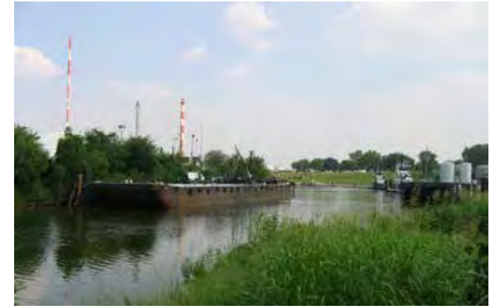
ABOVE: Photograph of Existing Conditions on Brady's Island BELOW, Left: Phytoremediation Process Diagram BELOW, Right: Marsh Ecology Section Diagram
