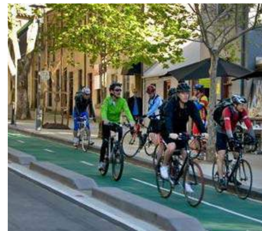
09 concrete bike lane delineators at intersection
