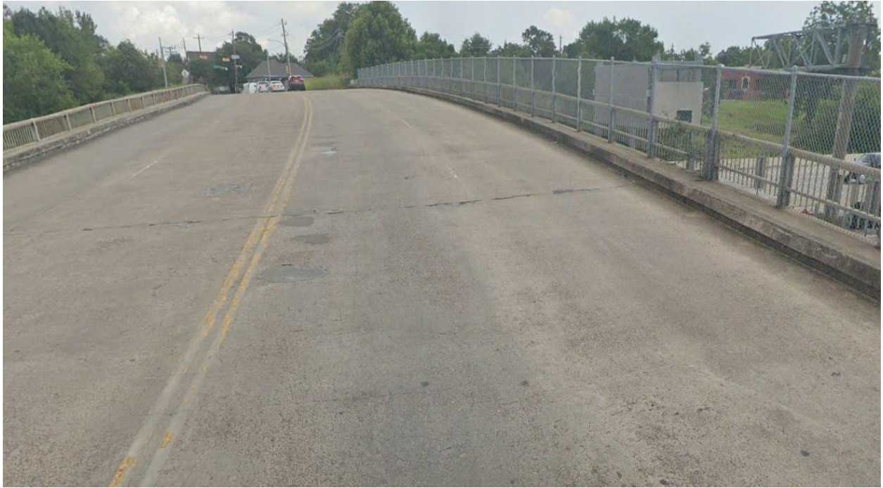
Quitman bridge over I45 looking east
