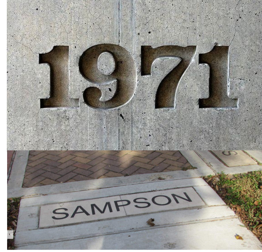
P.3 - INTEGRAL COLOR CONCRETE BAND W/STAMP - STREET NAMES
