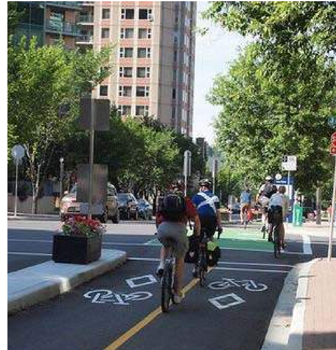
CONCRETE DELINEATOR AT INTERSECTIONS
