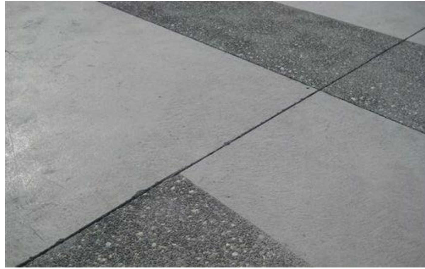
P.2 - UPGRADED CONCRETE PAVING - VARYING TEXTURES (SANDBLASTED & BROOM FINISHED SURFACES)
